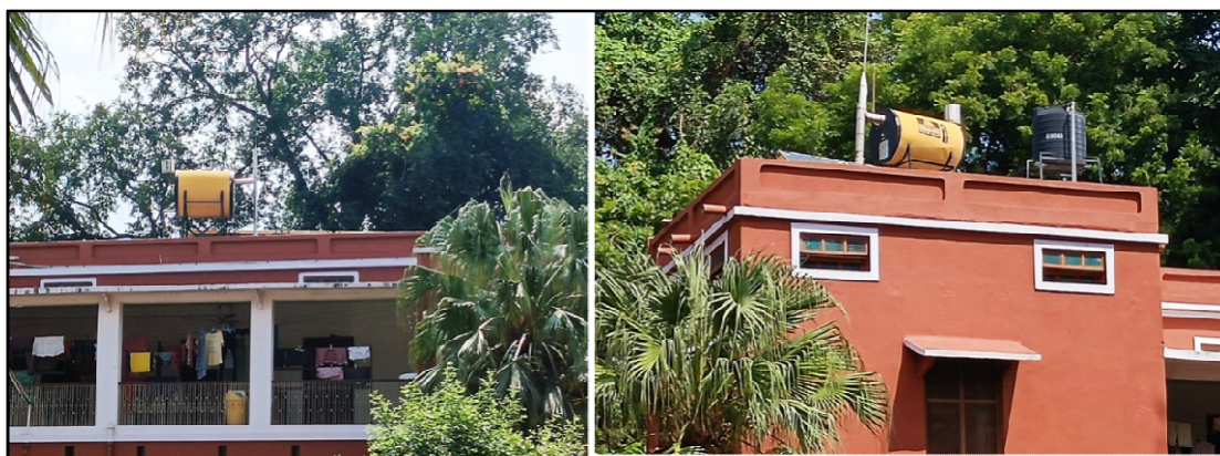
Figure: Rooftop solar heaters in hostels of VCW college
