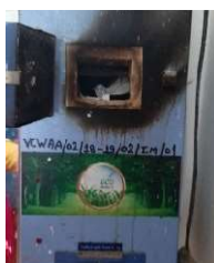
Figure: Sanitary napkin incineration machine installed in the washroom.
