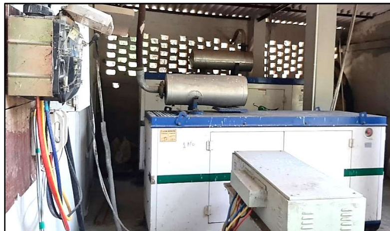
Figure : DG sets for Electricity Backup
