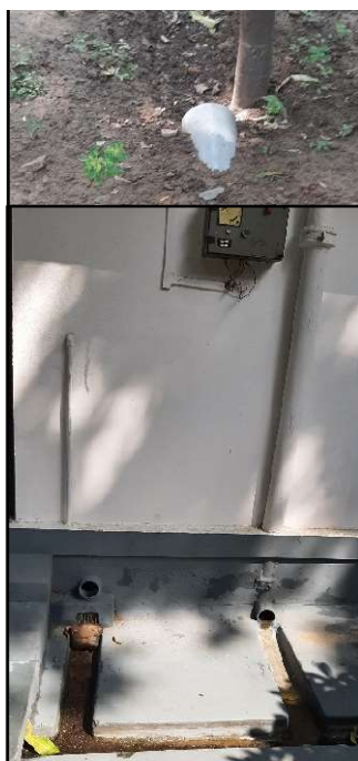
Figure: Water percolation from different buildings being utilized for gardening
