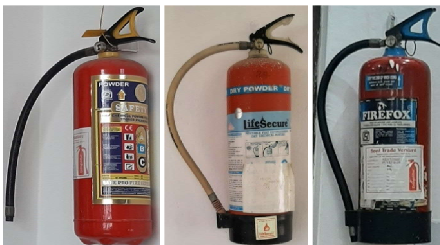
Figure: Fire Extinguishers installed at the campus premise
