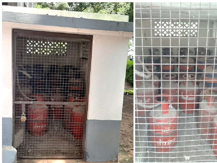
Figure: LPG cylinders housed separately in a storage shed outside the main campus building for safety
