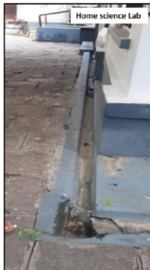
Figure: Effluent from home science lab is being channelized for irrigation purposes
